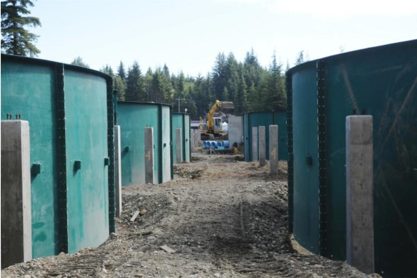
**The first module of the Namgis closed containment salmon farm includes five 500-cubic metre tanks and smaller tanks for quarantine of new smolts.**
